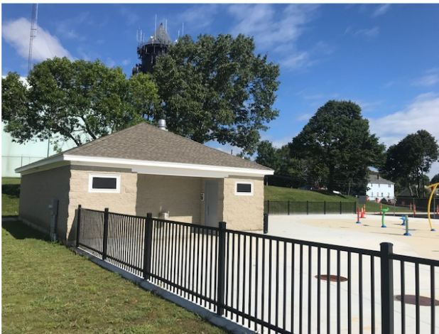
Splash Park Support Buildings
