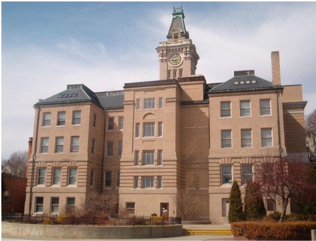
Envelope Restorations (window replacement and re-pointing)
