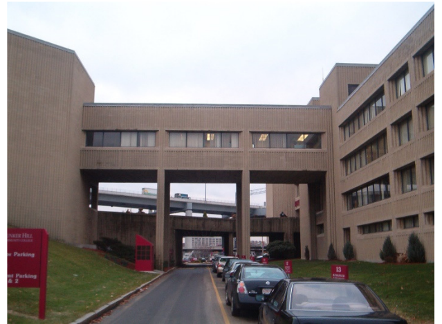
Envelope Restorations – Re-pointing and Repair
